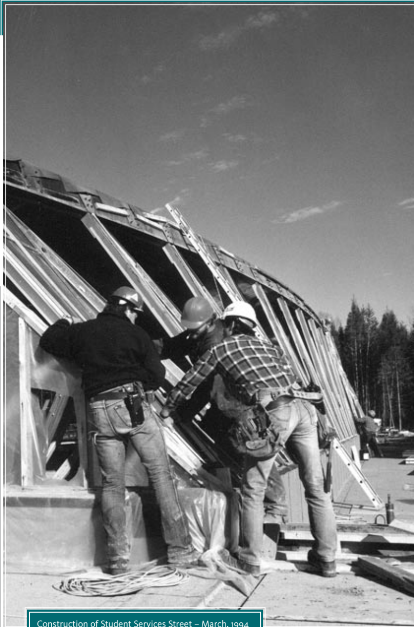
Construction of Student Services Street – March, 1994
